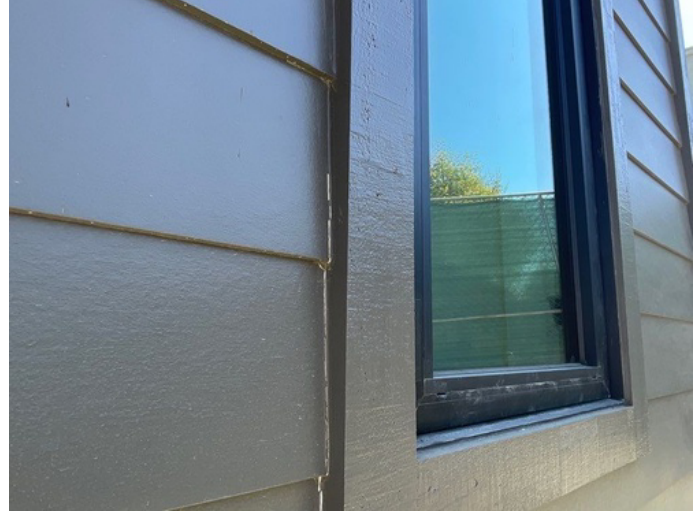
Includes adding/repairing caulking around windows and trim.
